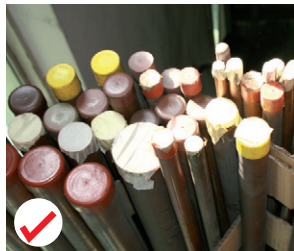
Piping materials are casually kept on the floor at a construction site. No seal plugs are placed on the ends of the tubes.
