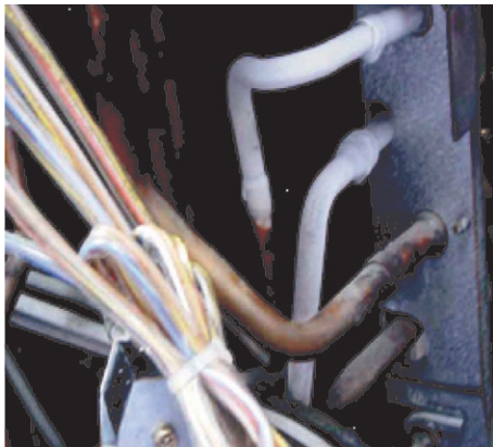
Frozen choke has occurred in the distributor on the outdoor unit heat exchanger.
